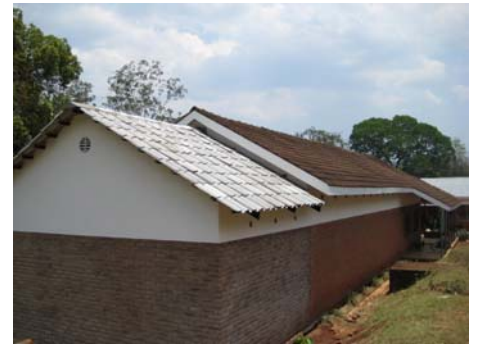
The pharmacy undergoing rehabilitation and extension. ▲
